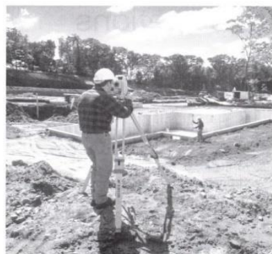
Measuring with a total station
