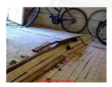
Extreme buckling can cause an upwards explosion of a wood floor when flooring is exposed to flooding or prolonged leaks.
