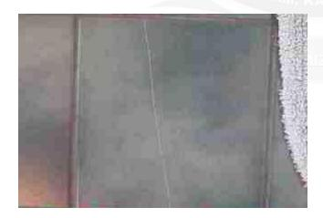
Cracked floor tiles like this can be diagnosed in order to decide if the cracking shows a serious structural problem, inadequate floor support, mechanical damage, or as in this case, damage from a loose, rocky toilet.
