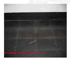
Asphalt floor tiles are 9" square (or other sized) tiles which used asphalt as the main binding material, the original asphalt tiles were produced only in dark colors because asphalt was a main ingredient.
