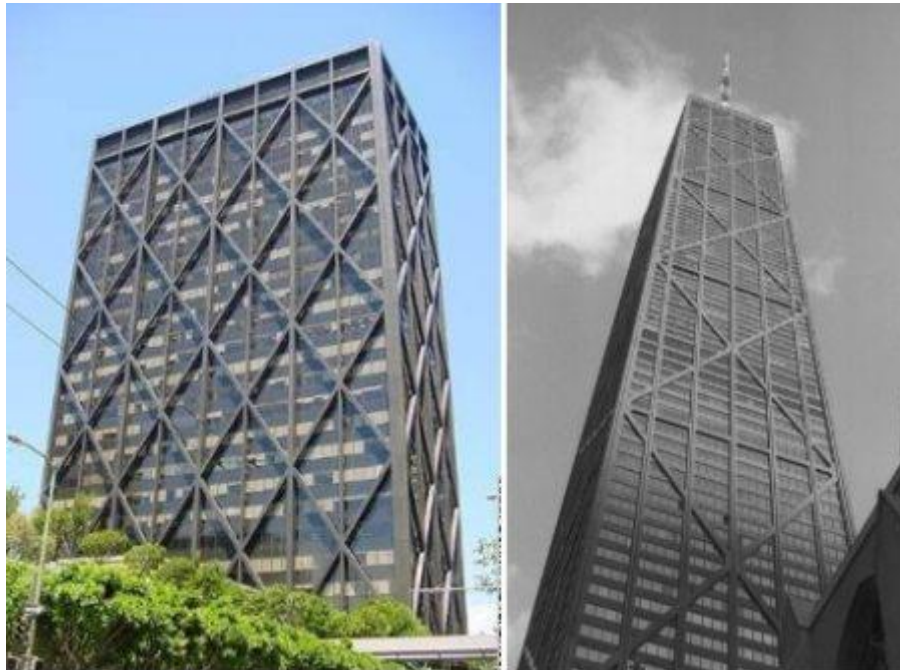
Fig.2: Braced frame structure
