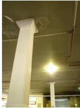
Fig.2.4. Flat slab without drop
