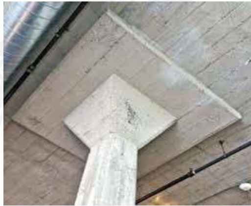
Fig.2.5. Flat slab with drop
