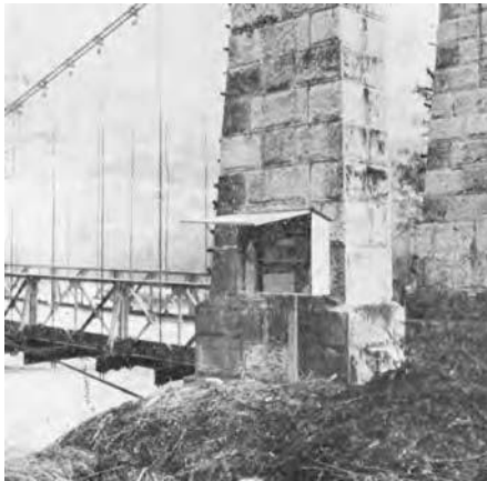
Fig. 5 Bubble Gauge Installation— Telemnip (Courtesy : Neyrtec, Grenoble, France)
