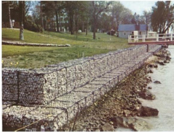
Bulkhead structure constructed by Gabion mesh boxes
