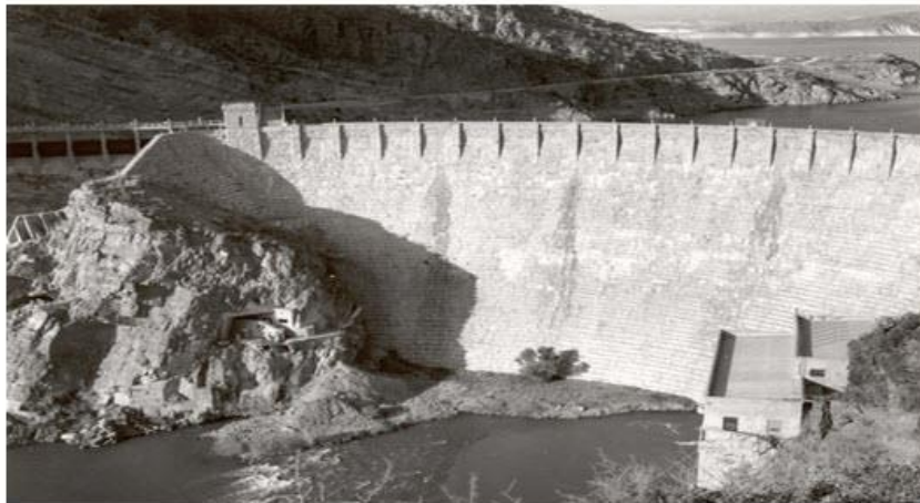
Fig. 31.1. Rubble-masonry gravity arch dam.
