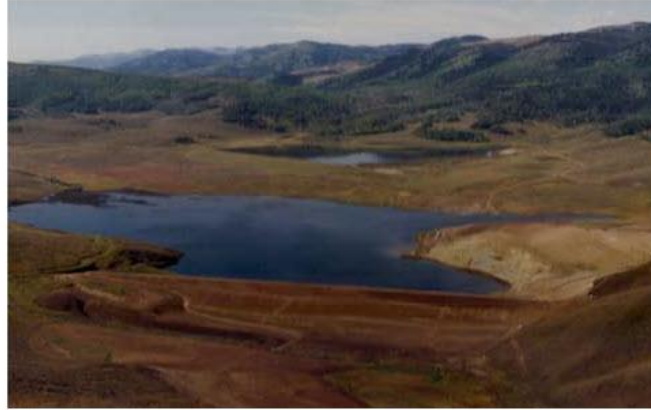
Fig. 31.7. Sand Detention Dam (Smoky canyon dam)
