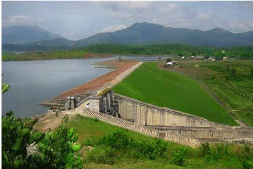
Fig. 32.4. The Banasura Sagar dam. (Source: http://www.banasura.com/banasura-sagar-dam )
