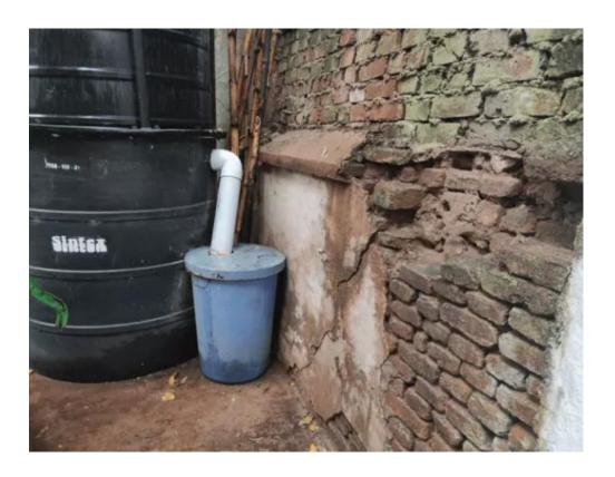
kitchen leftovers, cooked food, uncooked food, spoiled food, vegetable peels in the digester. The only catch is that the waste must be in liquid or semi-solid form. Therefore, it is better to either soak the waste or grind it in a mixie before feeding it into the digester. This is because the solid bits of waste may get stuck in the plant, hindering the biogas production.
