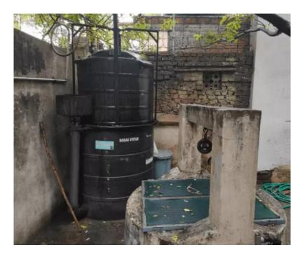
As biogas is produced inside the lower tank, it rises up to fill the gas storage container above, propelling it upwards.
