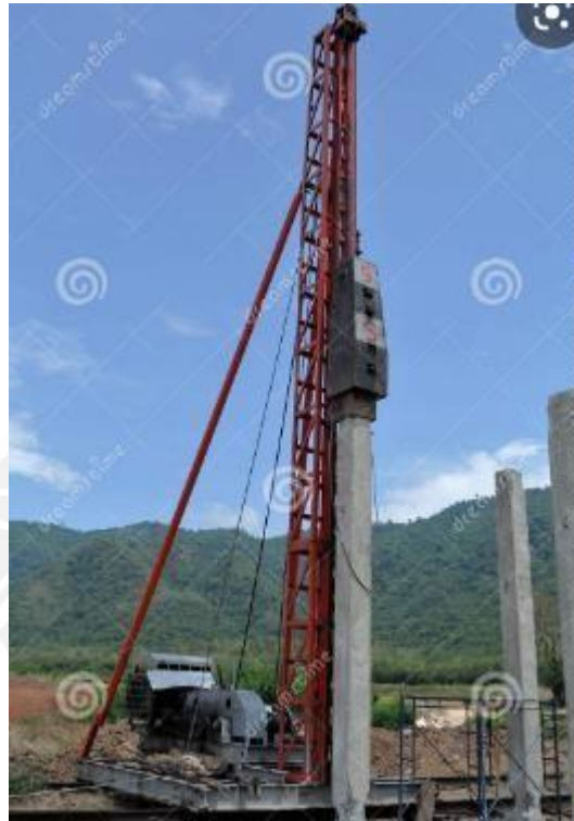
Figure-1: Pile driving using hammer
