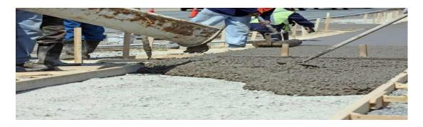
water should be adding in a measure quantity to obtain the design water cement ratio.
